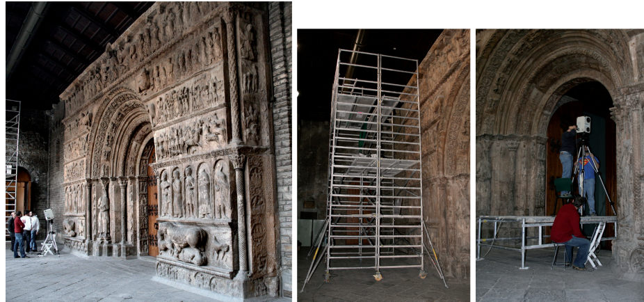
Fig. 1. The Portalada: Romanesque entrance of the Ripoll Monastery. Its size is clearly impressive as is the richness of the sculpted relief. Left: general view Middle: the 7 meter high scaffolding used for acquisition. Right: a smaller scaffolding used for the acquisition of the internal part of the portal.
